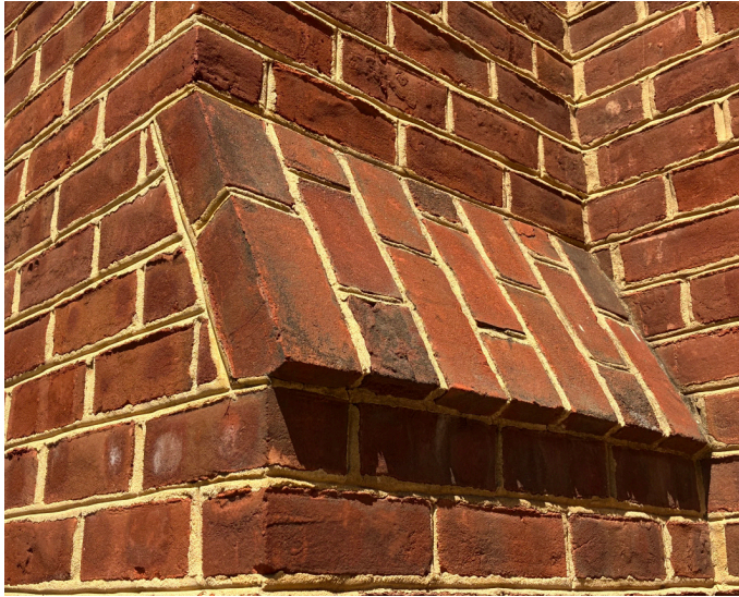
Figure 2: Chimney shoulder
